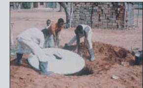
installation of a cover panel
