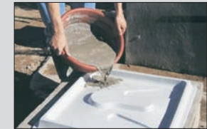
Making of a latrine slab
